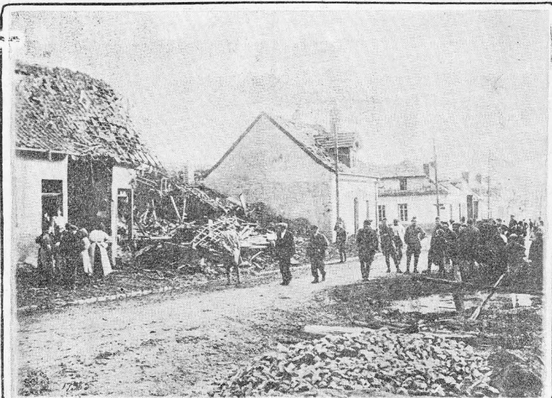
Buildings demolished by German air bombers, Beauval, July 14, 1918. 80th Divisional troops, stationed in the town, surveying the ruins.
