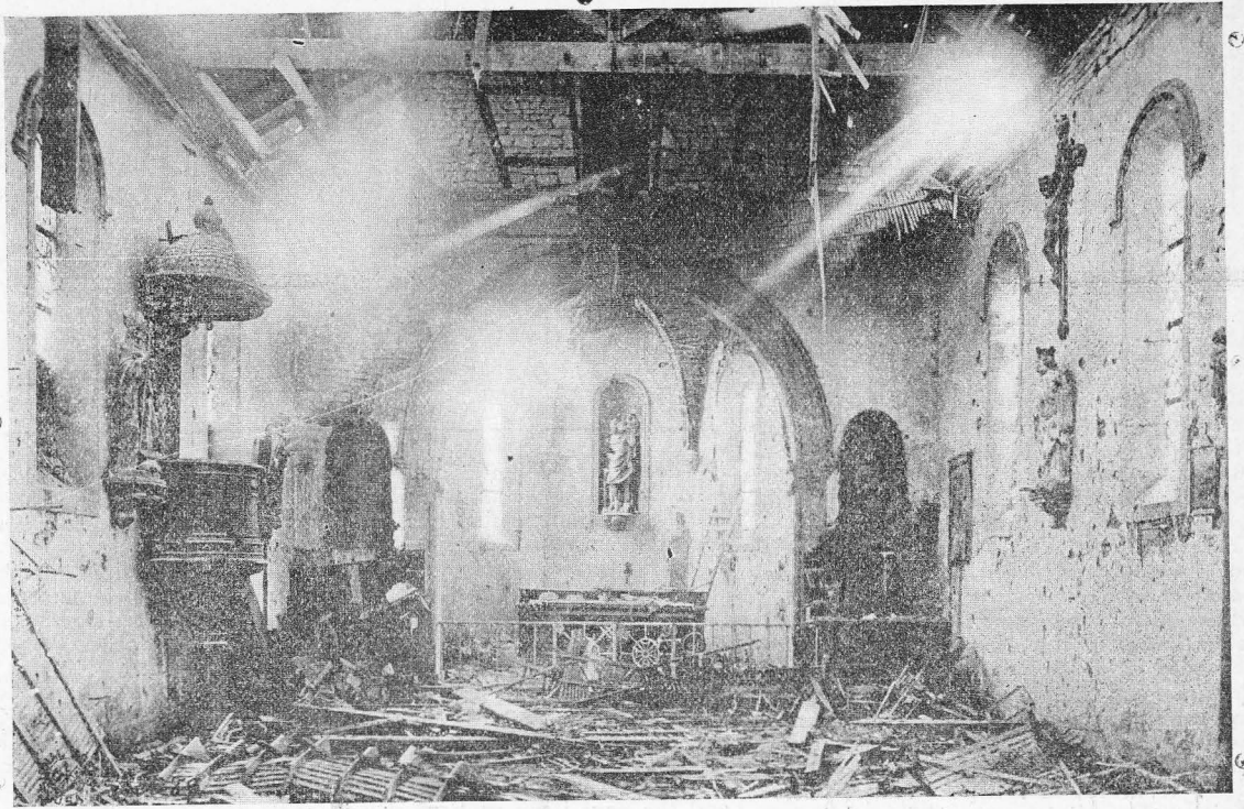
INTERIOR OF CHURCH AT CUNEL
