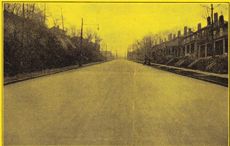
Section of Washington Boulevard, Pittsburgh, Pa., Laid with 'Colprovia'
