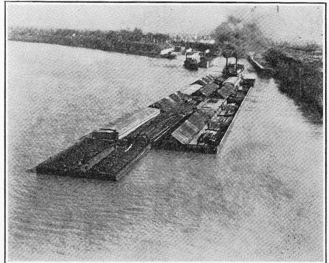
Coal Barge Fleet on the Monongahela
